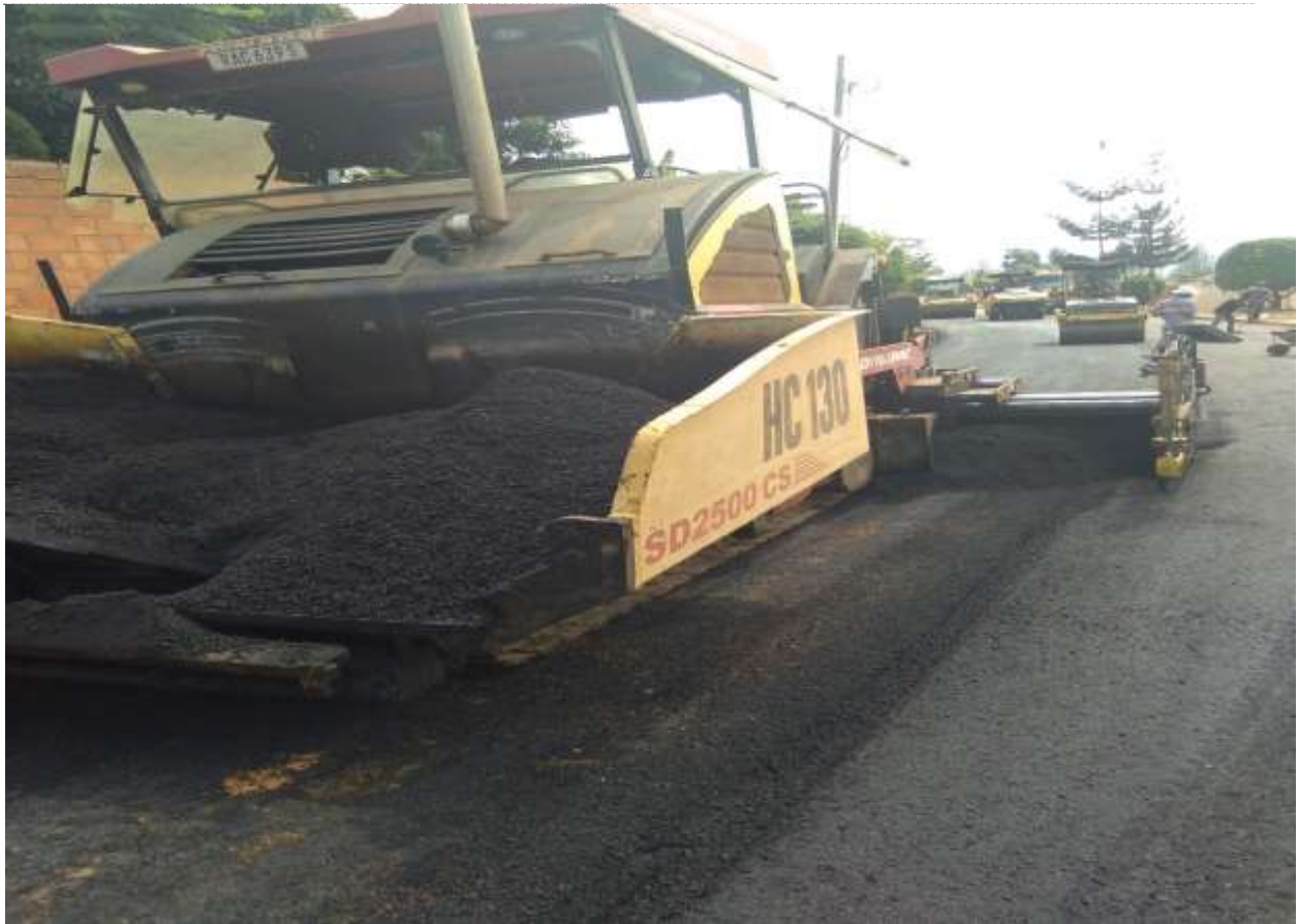
Picture8: Mobile asphalt layers and finishers
