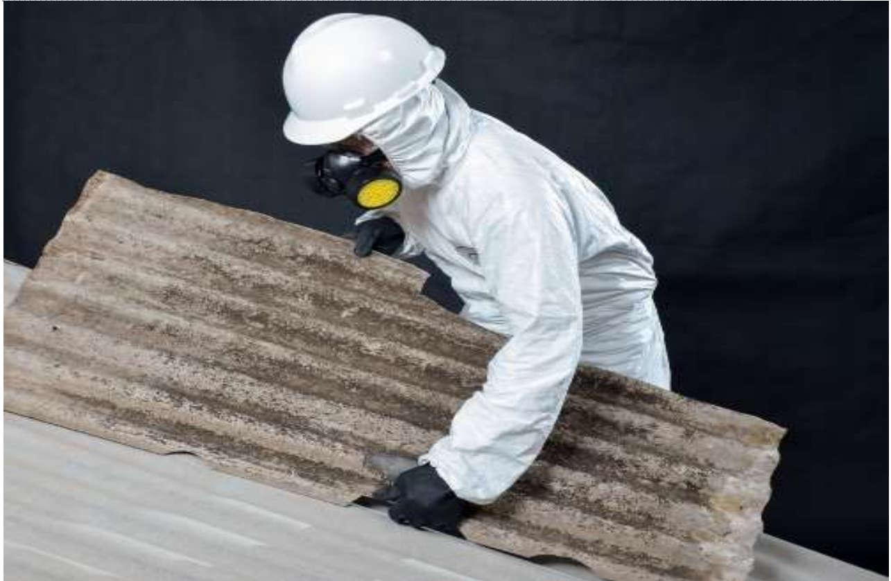
Picture16: Use and removal of asbestos protection equipment.
